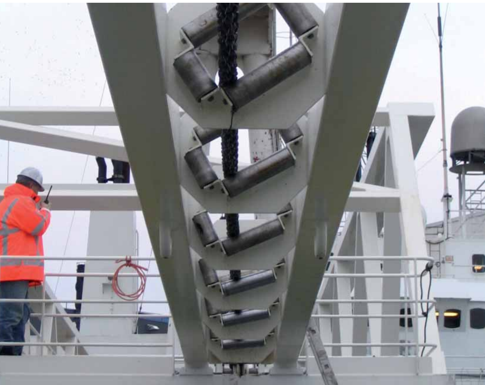
Cable transport system on the cable ship
